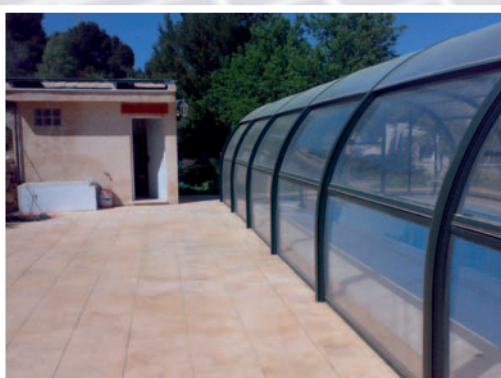
Solar pool heating in Muro (Spain).
